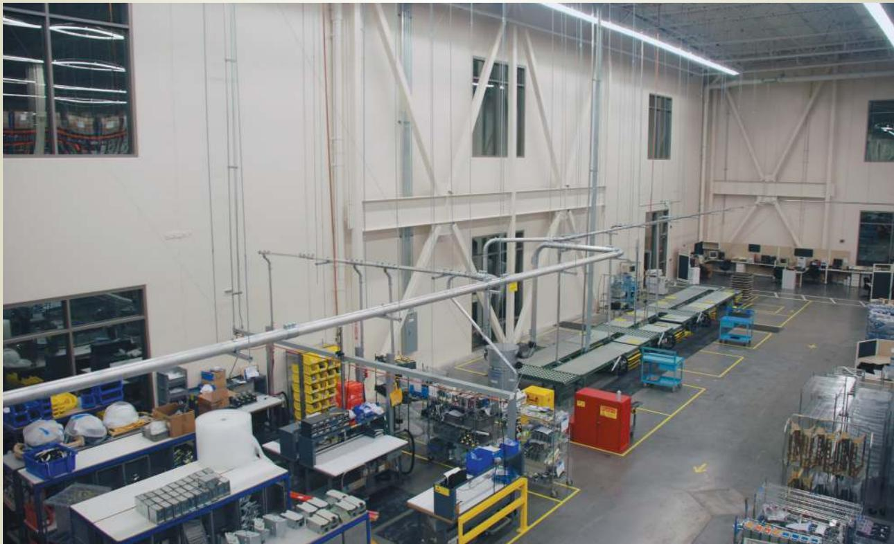
Your piping system delivers suction to the point of use, carries air and debris to your filtration devices, then returns clean dry air to the vacuum producer. Piping can have a dramatic effect on the overall performance of your vacuum system. Even the most powerful
