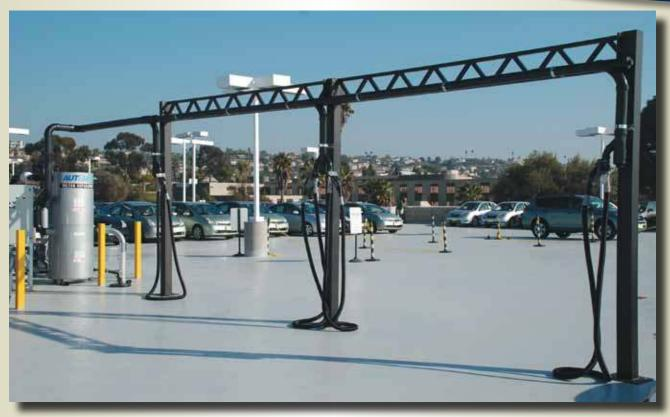
Your piping system delivers suction to the point of use, carries air and debris to your filtration devices, then returns clean dry air to the vacuum producer. Piping can have a dramatic effect on the overall performance of your vacuum system. Even the most powerful
